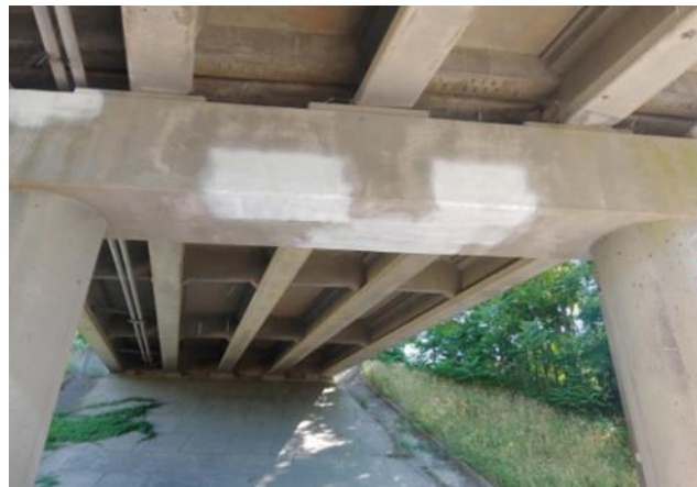
Figure 15. Condition after Remediation of Pier 1 of the Route 621 Bridge before Applying Epoxy Coating
