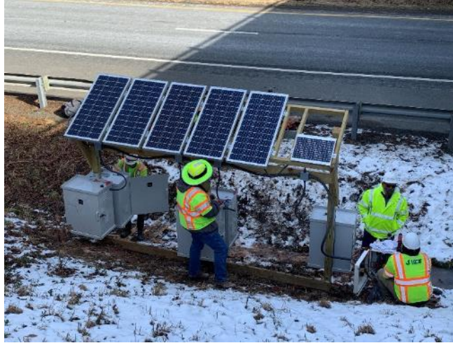
Figure 29. The Five Larger Solar Panels Supply Electricity for the Cathodic Protection System and the Smaller Solar Panel Powers the Remote Monitoring Unit
