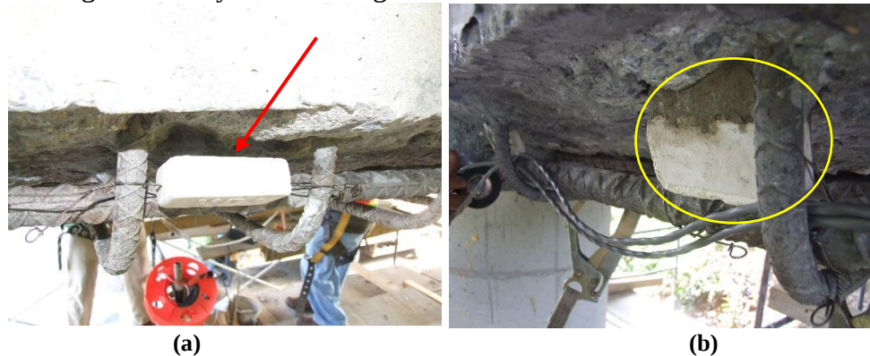
Figure 32. (a) Anode Installed along the Perimeter of the Repair without Embedment Mortar between the Original Concrete and Anode as Indicated by the Arrow; (b) Anode Installed with Embedment Mortar (top of yellow circle) to Enhance Current Flow to the Original Concrete
