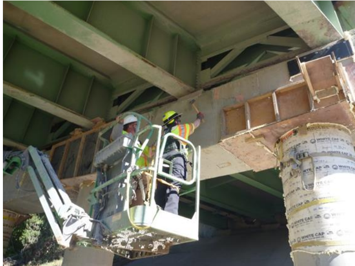
Figure 25. Route 605 Bridge over I-64 (Columns and Pier Cap along Westbound Lane). After the removal of forms, the area was tapped with hammer to determine if the repairs were sound.
