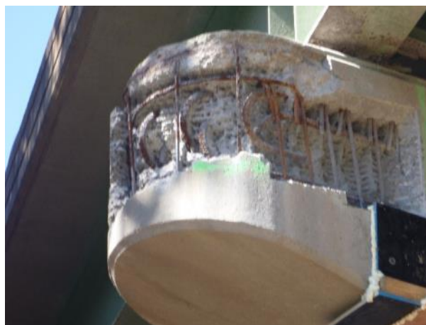
Figure 24. Rout 605 Bridge over I-64 (Pier Cap along Eastbound Lane). Concrete removed from the end of a pier cap using hydrodemolition. The area must be pressure washed to remove the cement slurry left after hydrodemolition.
